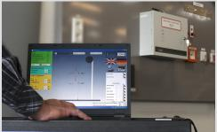
SKC-SC controls fire curtains and smoke curtains. It has been tested in accordance with prEN 12101-9 and BS 8524. It has a power supply to maintain the control functions for at least 72 hours in accordance with EN 12101-10.
