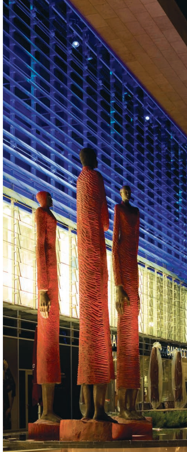
Alstertal Shopping Centre in Hamburg. 809 coloured back-lit adjustable glass louvres emphasize the living character of the urban quarter
