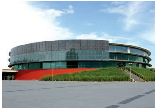
EWE Arena, Oldenburg, Germany. The defining feature of this stadium is a moveable glass panelled solar shading device which is fitted with photovoltaic cells. The curtain walling comprises 6m high photovoltaic solar shading panels which track the sun as it moves around in the sky. The whole installation measures 40m long.
