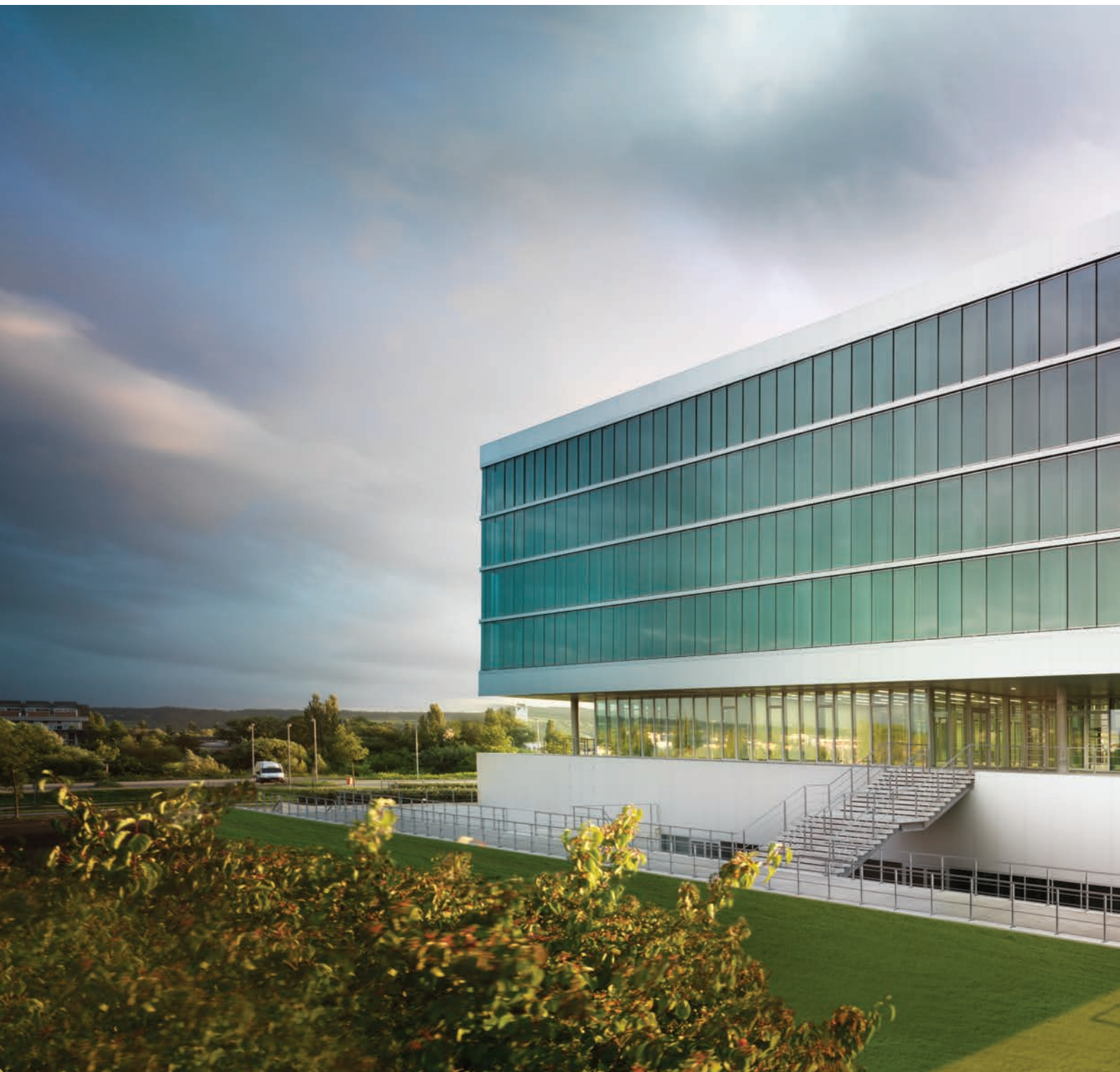
Nycomed Office Building in Konstanz, Germany. Impressive visual appeal combined with excellent performance. The building envelope consists of an active façade consisting of moveable glass louvres which provide solar shading and defence against inclement weather. The glass louvres have a 60% frit to reduce the solar heat gain but allow enough light to come through. The blades are continuously moving to their optimum positions and those inside keep an excellent view to the exterior.
