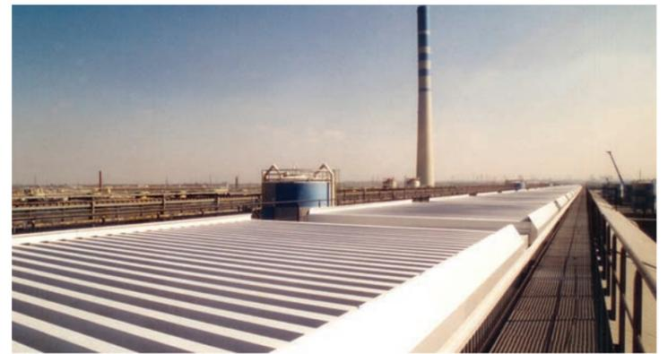
In 1980 Colt was required to replace existing mechanical HVAC equipment at Trimet aluminium in Essen, Germany in response to changing needs, and supplied a scheme of natural/gravity ventilation. This scheme consisted of a Labyrinth Ventilation system and wall louvres. Now, after more than 30 years of operation the system is still in a very good condition and shows no sign of destructive corrosion.
