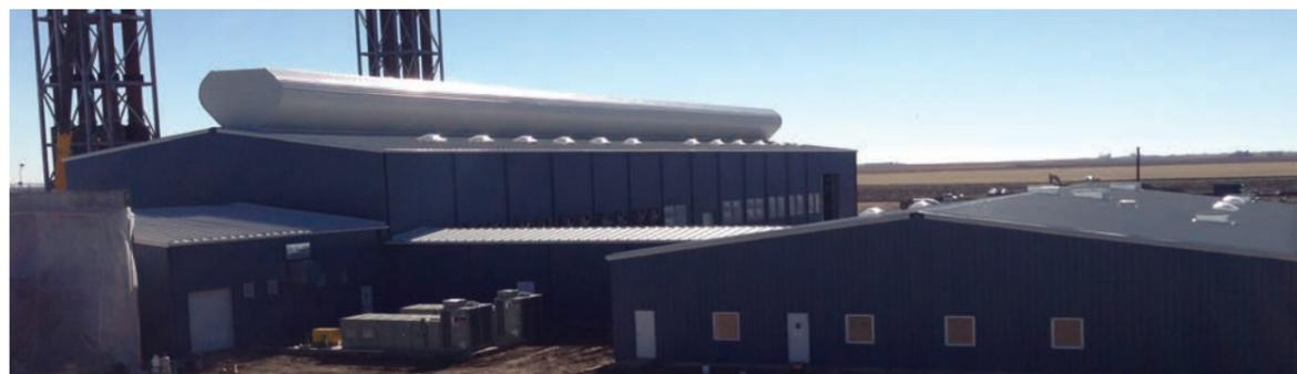
A scheme of MoffittVent ventilators measuring 288" x 108" (88m x 7.3m) is being installed at this new facility. These ventilators include 6 motorized dampers so as to shut off the units when they are not in operation.
