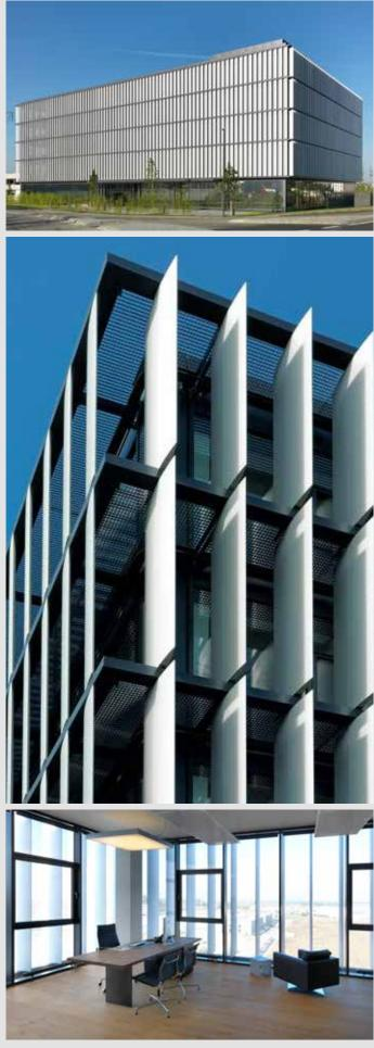
The facade elements ensure optimum levels of daylight and reduction in cooling loads whilst providing a striking aesthetic.
