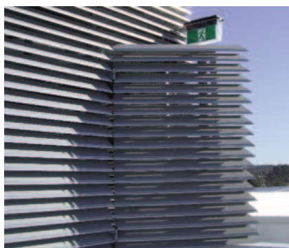
University of Western Sydney, Parramatta, New South Wales. PR100 Louvre door, in open position.
