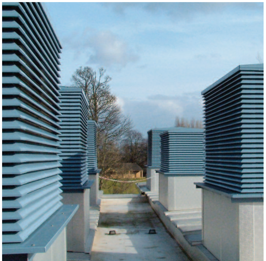
Pre-assembled 3UL louvre turrets on top of natural vent shafts.
