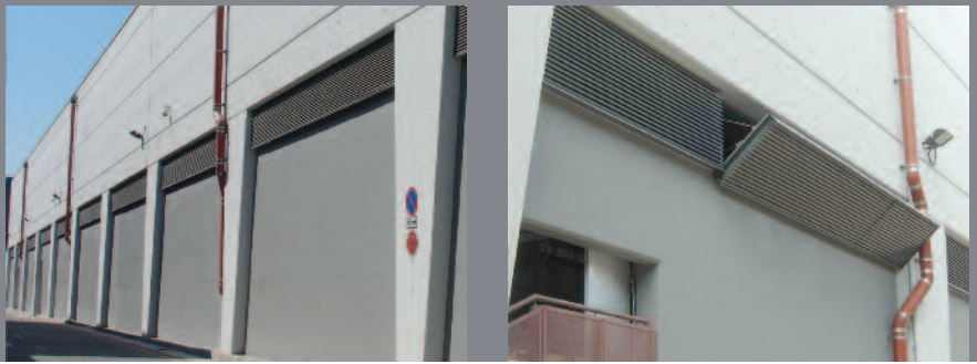
Side vents fitted externally with Colt Universal Louvre in line with surrounding Colt Louvre panels.
