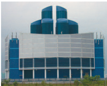
Triple bank faceted circular louvre installed to handle the high air volumes required and to provide maximum rain protection even in typhoon conditions.
