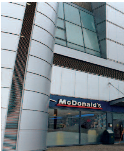
2000m 2 of Universal Louvre including both Colt Single Bank and Double Bank Universal rain defence louvre.
