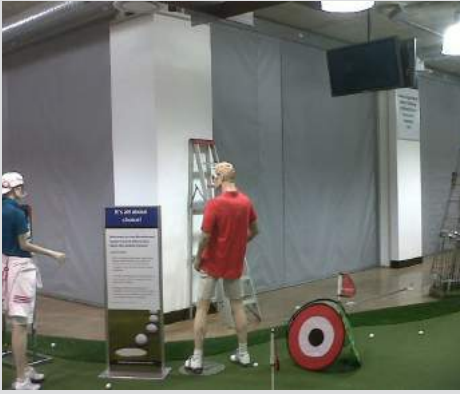
Retail - fire curtain lowered
