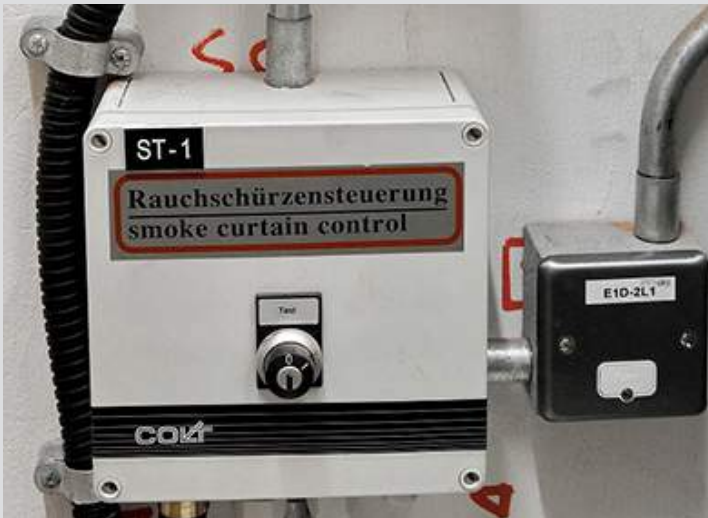
Set up for Option 1 controls (showing them installed on a project)
